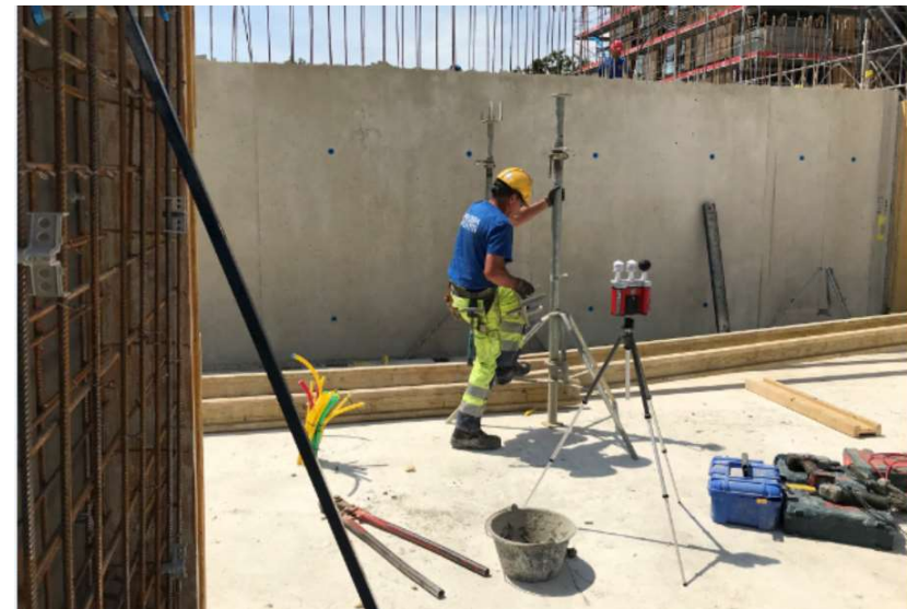
Preparation of slab formwork base
